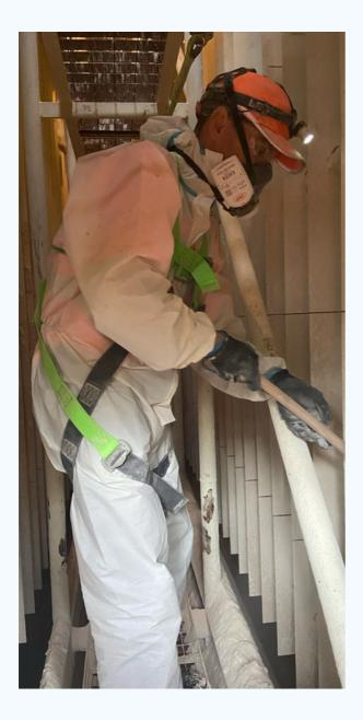
Regular cleaning of ESP and Luhr bag filter plants is essential for their regular upkeep and maintenance. However, this is a **highly specialised service** as projects are often constrained by **tight shutdown deadlines and company inspections.** If the project runs over time or is not completed to a high enough standard, you can face costly fines or damaging inspection failures.
